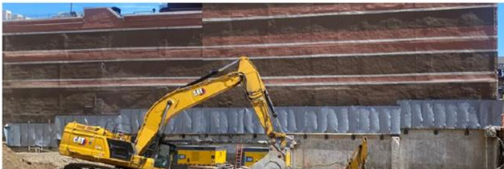
Sound blankets installed in front of Chung Pak Building. 松柏大廈前方待安裝隔音毯之區域。
