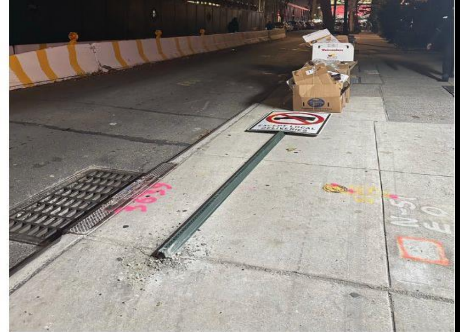
The sign was run over by a truck driver within a day of installation. Photo: Block Association
