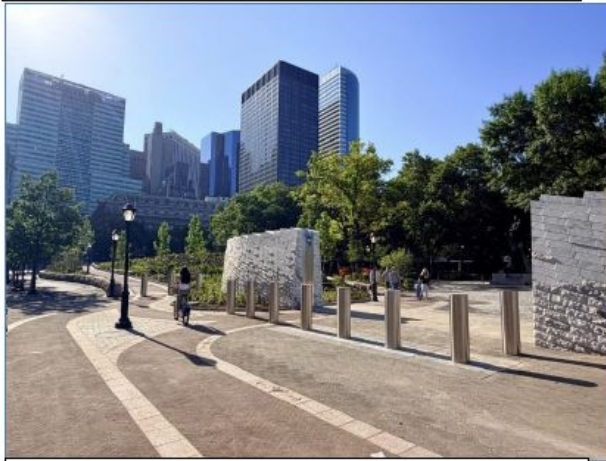
Stone floodwall and bollards
