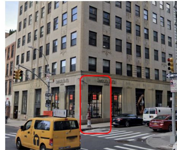
④ AREA OF WORK IN THIS APPLICATION Photo taken at intersection of Church Street & Franklin Street
