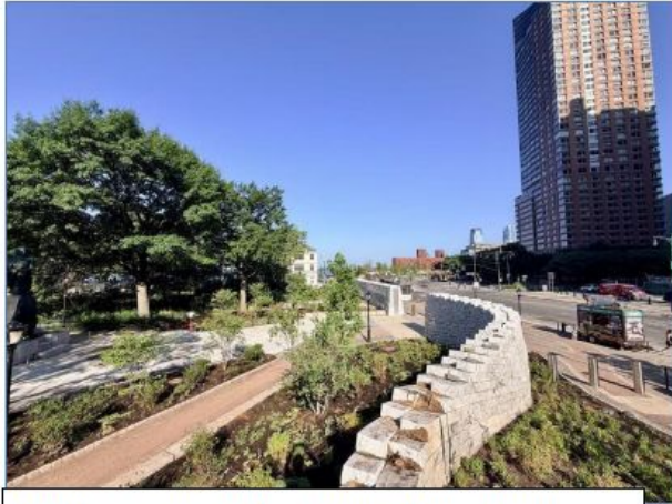
Northern edge of The Battery along Battery
